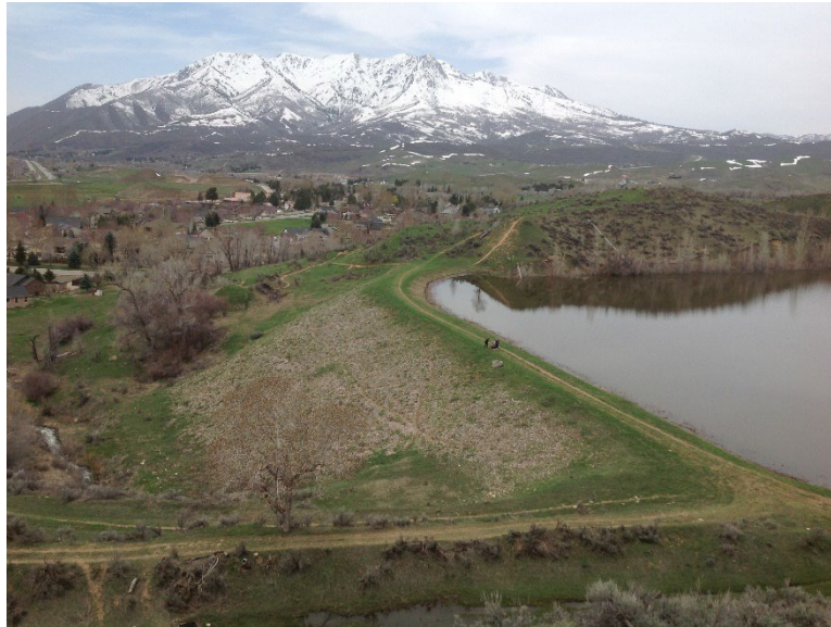
Caption: General overall view of dam embankment.
