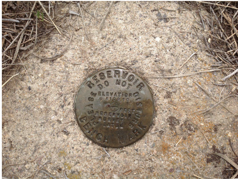
Caption: Close-up view of left (east) abutment benchmark (BM #2).
