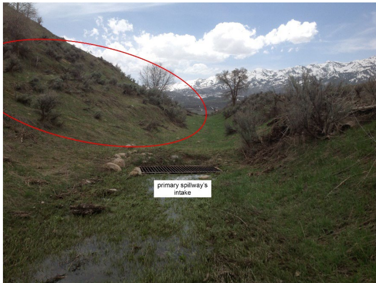
Caption: Historic landslide in the emergency spillway discharge channel.
